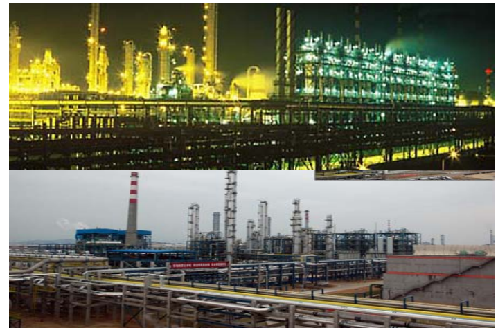
Yangtzi Petro-chemical Plant
