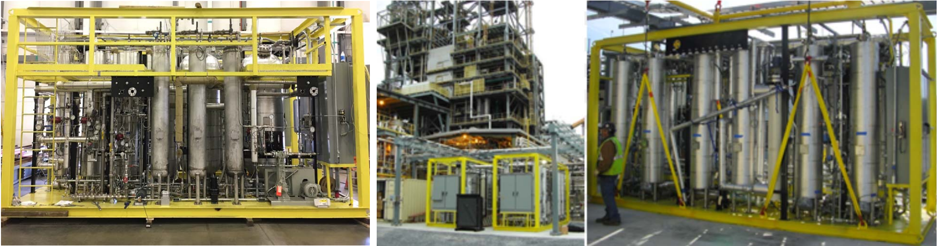
TDA 0.1 MW pre-combustion carbon capture unit installed at the National Carbon Capture Center
